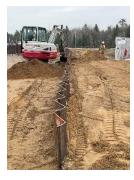
The sheet pile is nearing completion on the West side of Secord dam to the shore.
