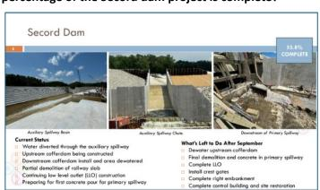
The Secord dam restoration project is about 56% complete. The estimated cost is \$66 Million with \$50 Million projected to be spent prior to the suspension in September.
